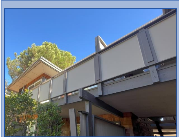
Underside of balcony is in good condition
