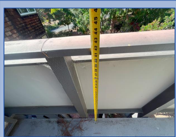
Railing height meets current building code requirements
