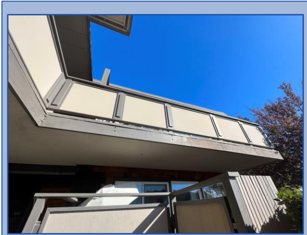
Underside of balcony is in good condition
