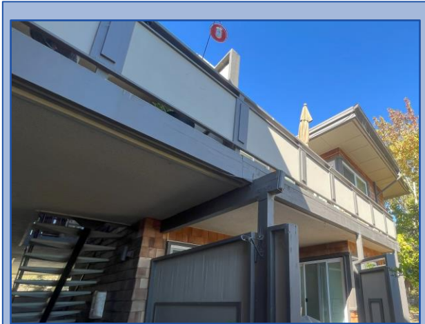
Underside of balcony is in good condition
