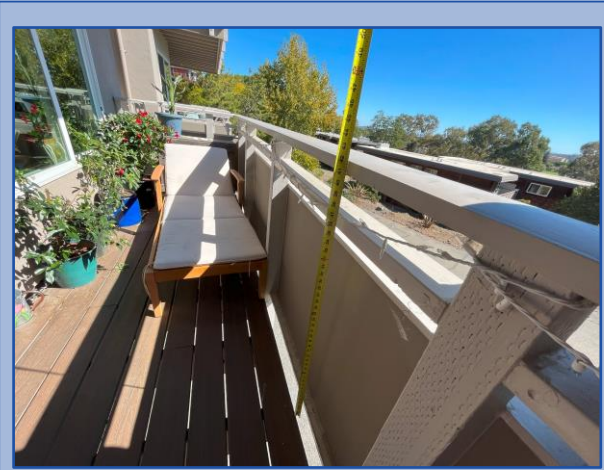
Railing height meets current building code requirements
