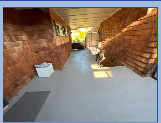
Walkway surface is in good condition
