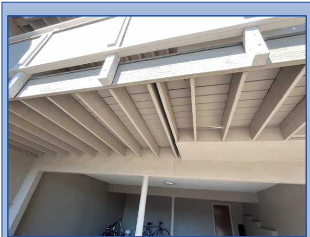
Underside of balcony and framing are in good condition
