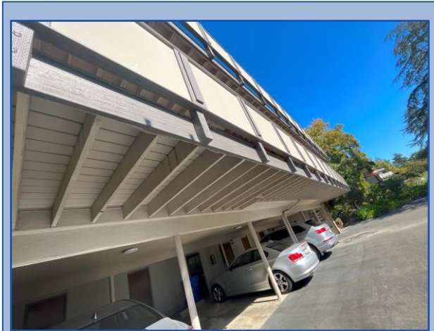
Underside of walkway and framing is in good condition
