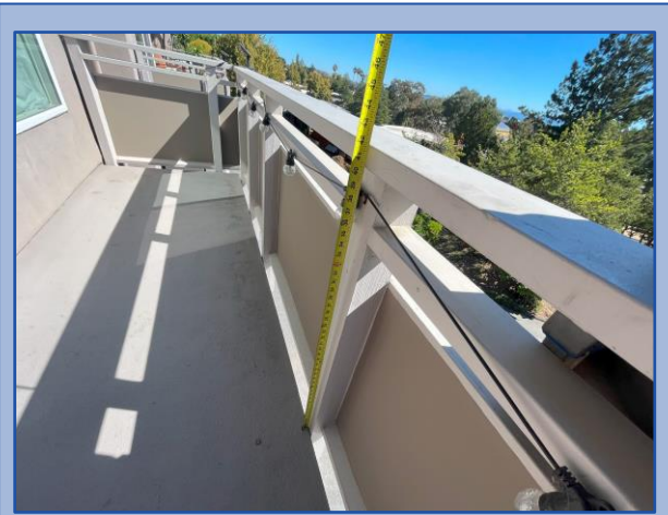
Railing height meets current building code requirements
