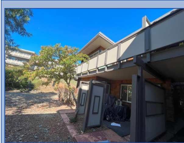
Underside of balcony is in good condition
