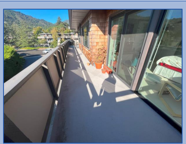
Walkway surface is in good condition
