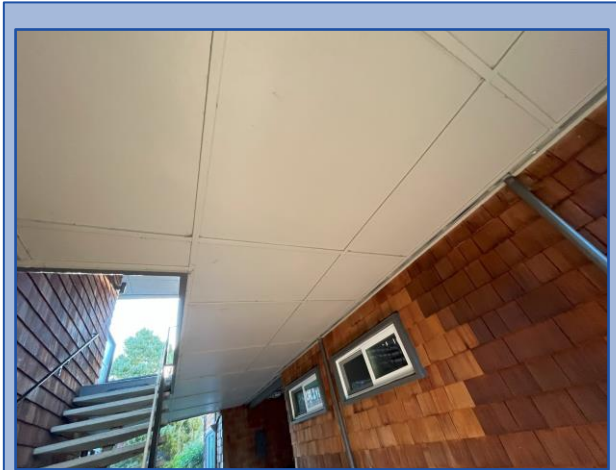
Underside of walkway is in good condition
