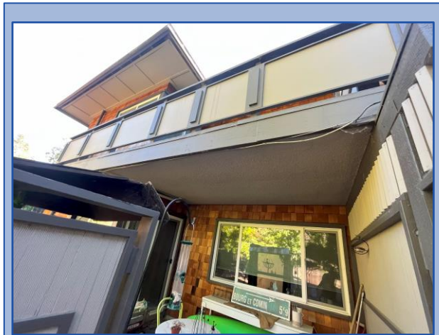
Underside of balcony is in good condition
