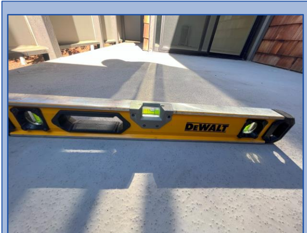
Balcony surface is properly sloped to encourage drainage
