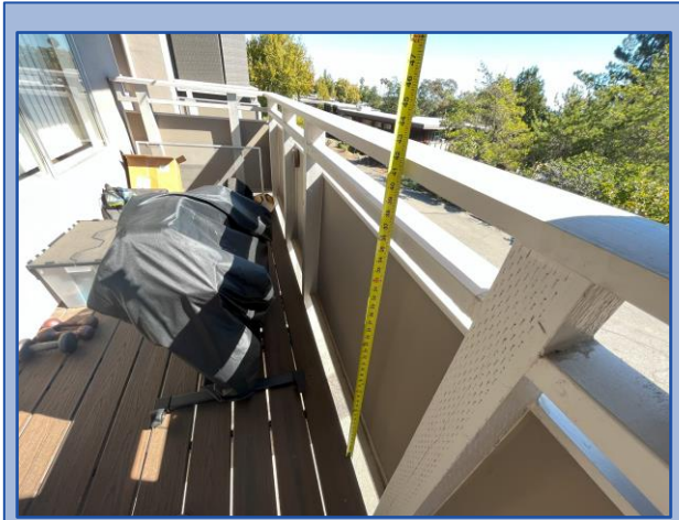
Railing height meets current building code requirements
