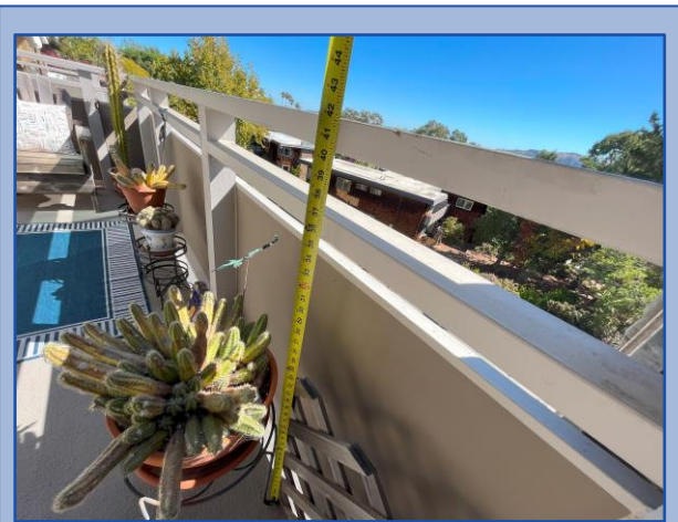
Railing height meets current building code requirements
