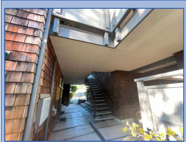
Underside of walkway is in good condition
