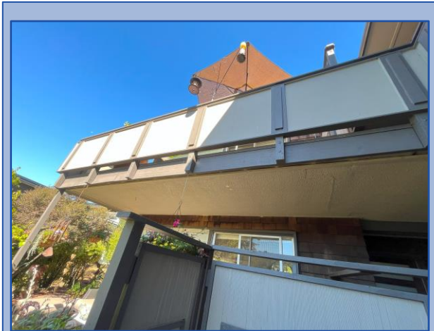
Underside of balcony is in good condition
