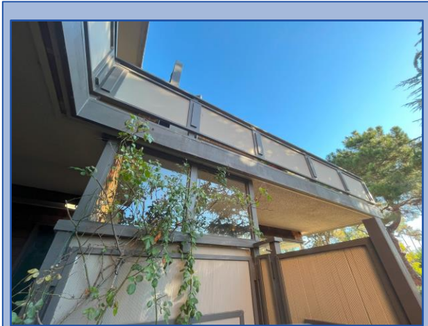
Underside of balcony is in good condition
