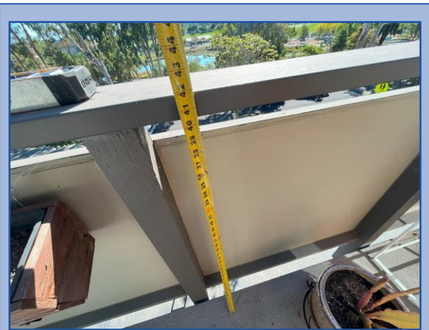
Railing height meets current building code requirements
