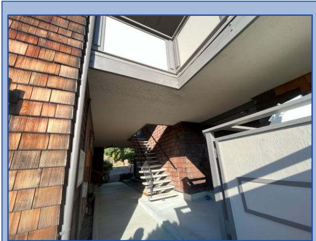
Underside of walkway is in good condition
