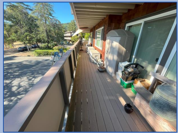
Walkway surface is in good condition
