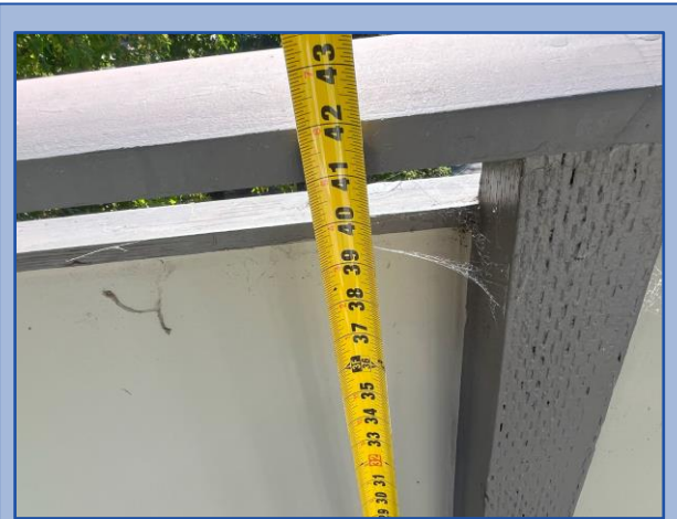
Railing height meets current building code requirements
