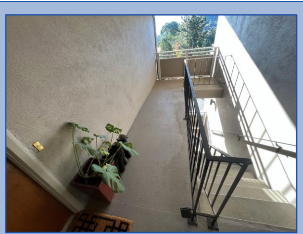
Walkway surface is in good condition
