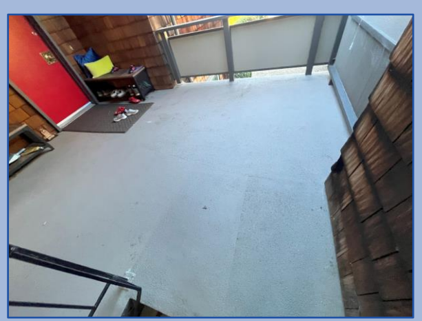
Walkway surface is in good condition
