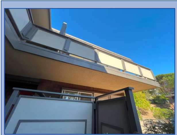
Underside of balcony is in good condition
