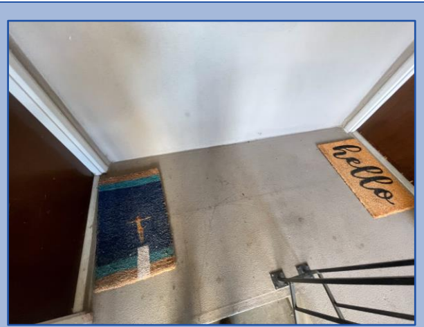
Walkway surface is in good condition
