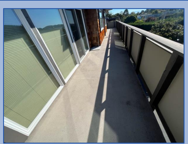
Walkway surface is in good condition
