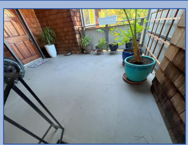
Walkway surface is in good condition
