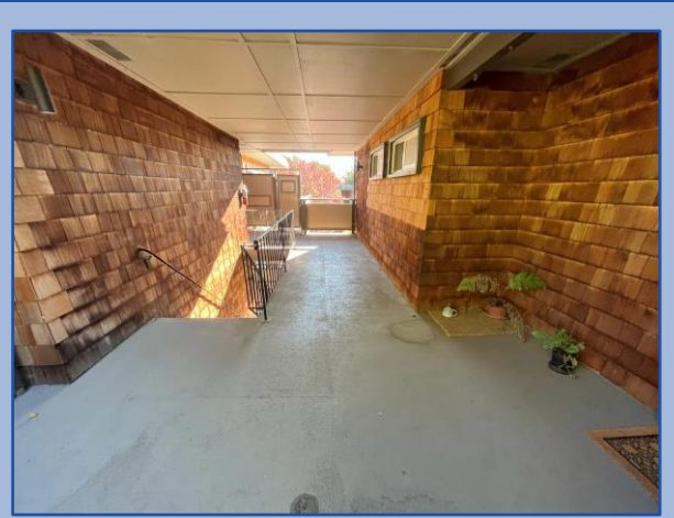
Walkway surface is in good condition
