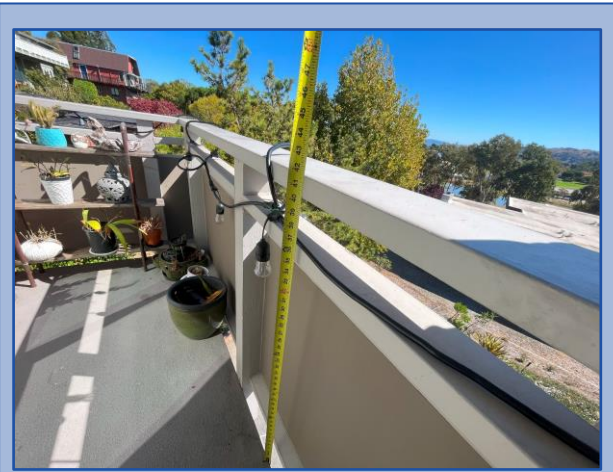
Railing height meets current building code requirements
