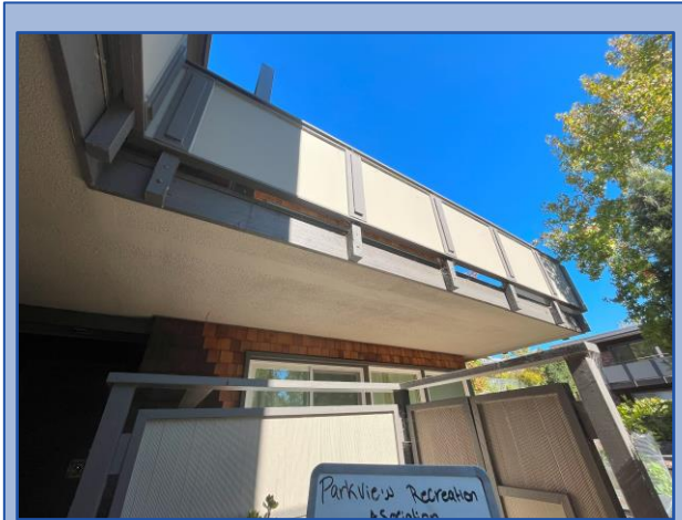
Underside of balcony is in good condition
