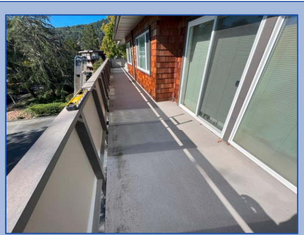
Walkway surface is in good condition
