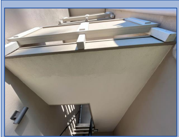
Underside of walkway is in good condition
