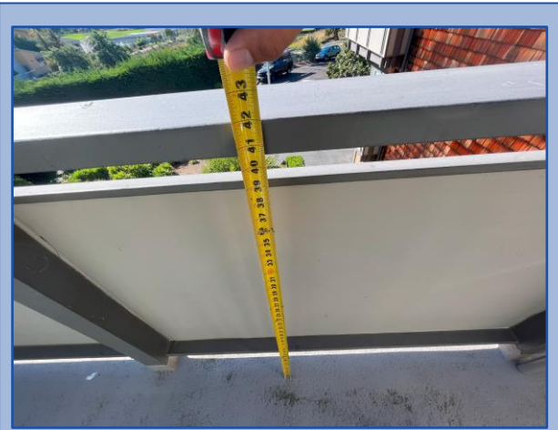
Railing height meets current building code requirements
