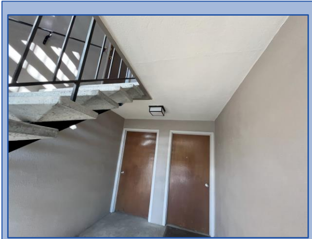
Underside of walkway is in good condition
