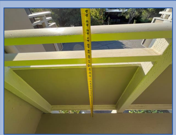
Railing height and baluster spacing meet current building code requirements
