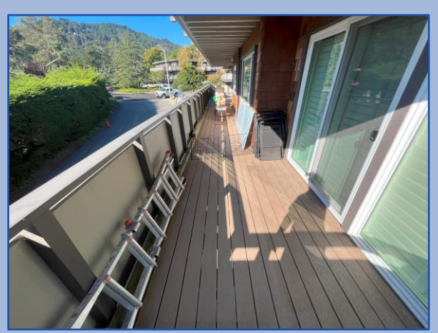
Walkway surface is in good condition
