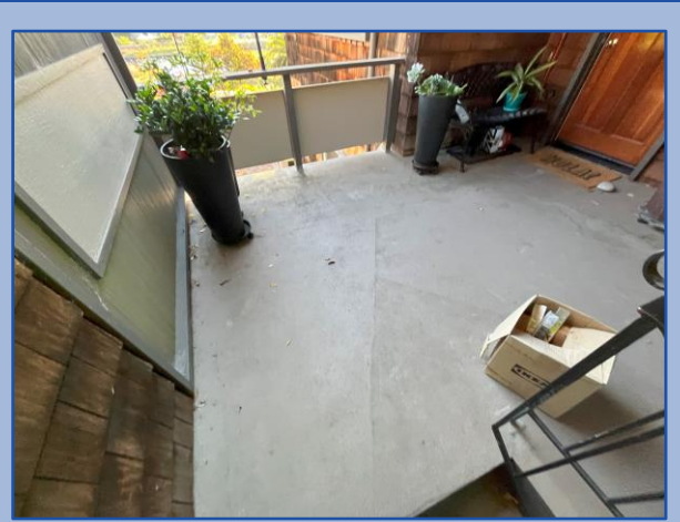
Walkway surface is in good condition
