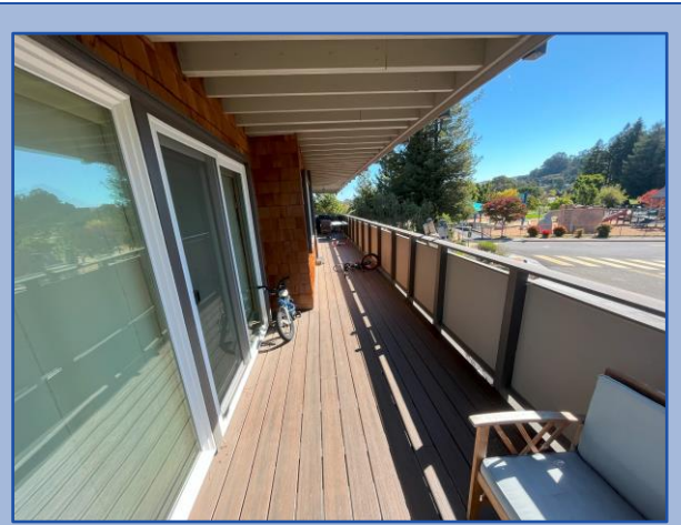
Walkway surface is in good condition
