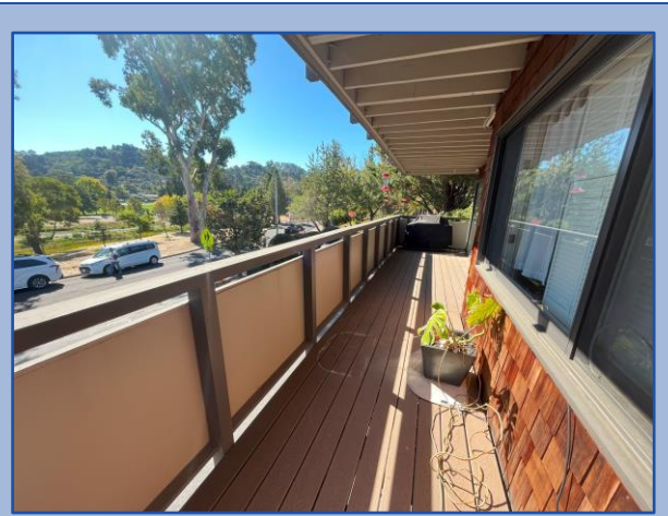
Walkway surface is in good condition
