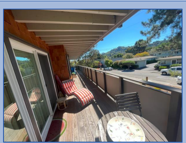
Walkway surface is in good condition
