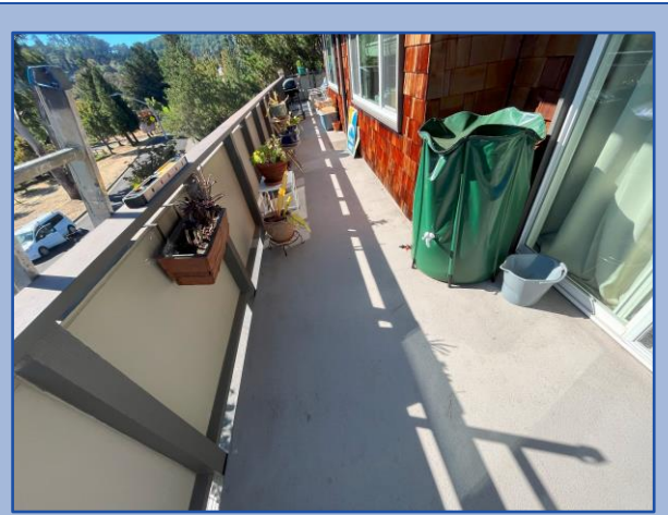
Walkway surface is in good condition
