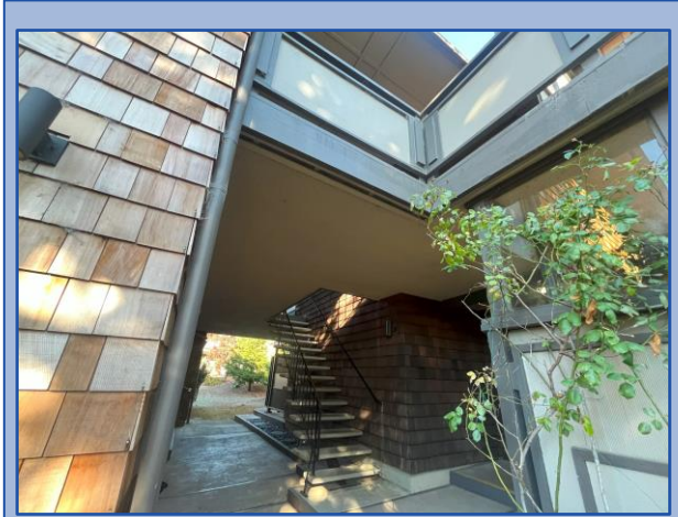
Underside of walkway is in good condition
