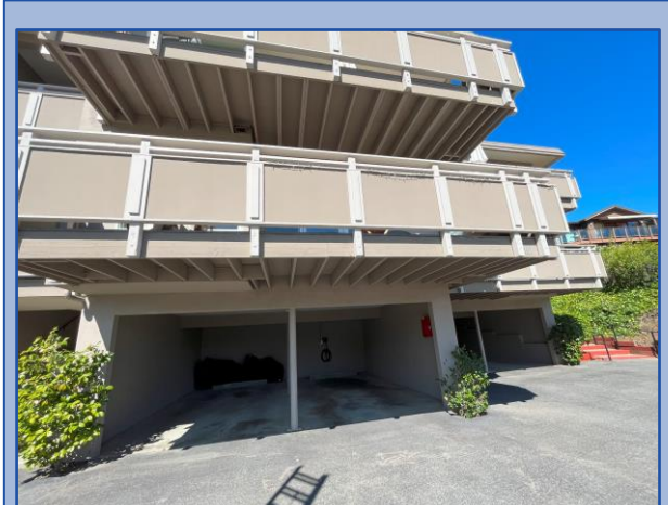
Underside of balcony and framing are in good condition
