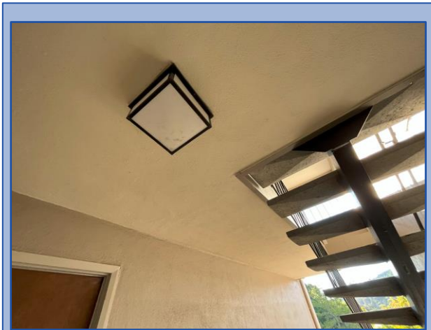
Underside of walkway is in good condition
